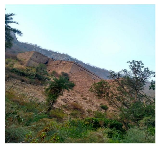
Figure 11: Side view of the 3 storeys, the top 4 have collapsed
